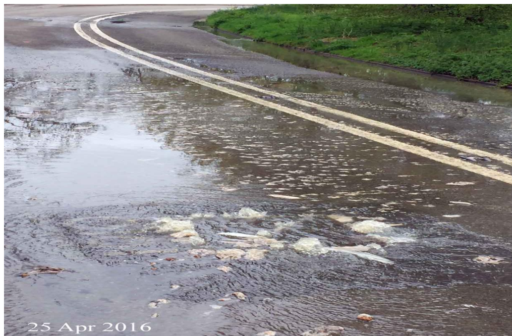
Image 3: Overflowing sewer on 'Old' Maidenhead Road April 2016
