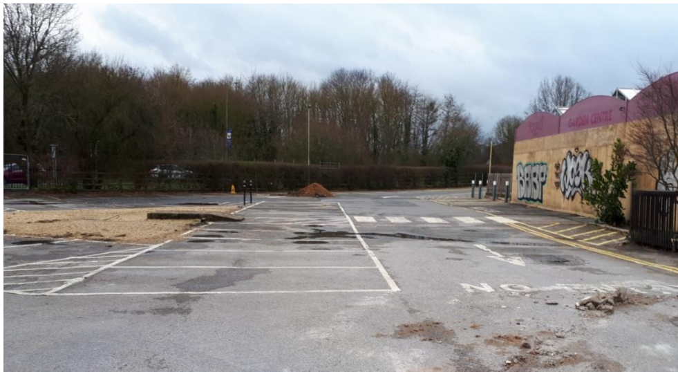
Image 1: Part of Application Site within Flood Zone 1, Saturday 26 January AM, following ~20 mins light drizzle. Standing water is visible.
